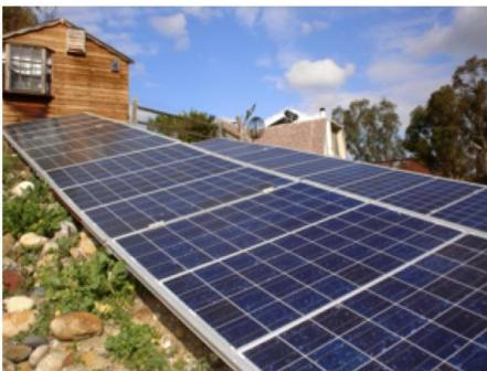
*Multicrystalline 2.8 kW, the Phase 2 is ground-mounted.*
