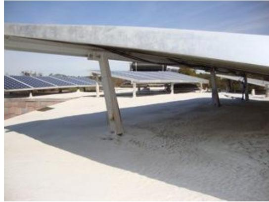
After the [rooftop PV](#) & solar hot water in 2003, we installed foam on our flat rooftop. This white foam reflects sun in Hot Summers helping cool our building, and is an insulator in Winters like snow helping hold in warmth. This is reducing energy use year-round. Moreover it is keeping rain from seeping through the flat roof, a side benefit.
